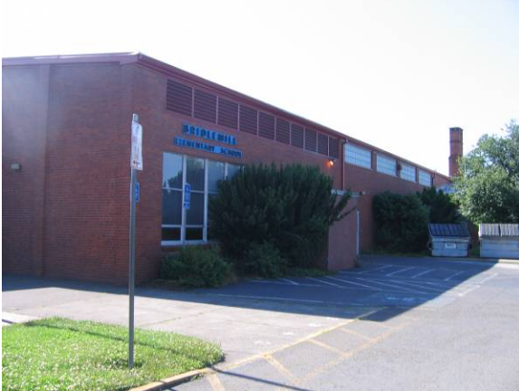
West elevation facing southeast
