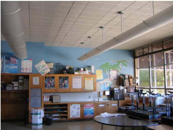
Classroom facing north
